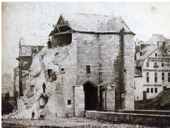
The porte de Louvain during its demolition in 1862.
